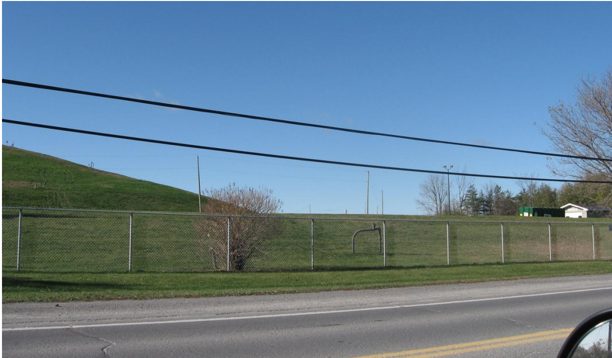
Photo 13. Carp Road north of Highway 417 – looking northwest to the landfill site. Fully exposed view of the Preferred Landfill Footprint.
