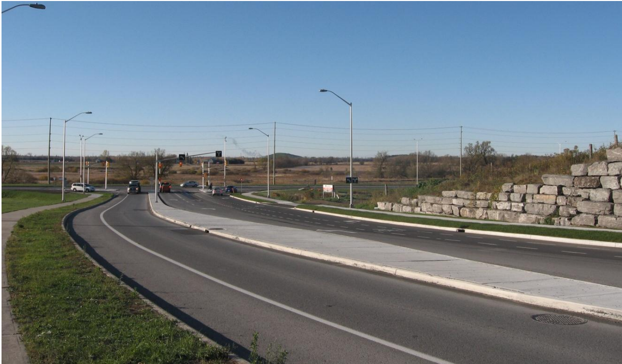
Photo 1. Kanata Avenue east of Terry Fox Drive – looking west to landfill site. Partially screened view of Preferred Landfill Footprint.
