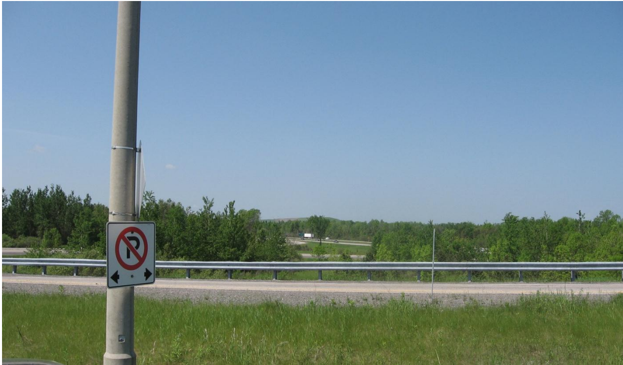
Photo 17. Huntmar Drive at Highway 417 – looking west to the landfill site. Partially screened view of the Preferred Landfill Footprint.
