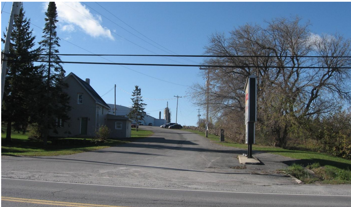
Photo 14. Carp Road at Laurysen Kitchens – looking west to landfill site. Partially screened view of the Preferred Landfill Footprint.
